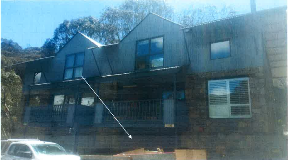
Figure 2: Materials can be stored within the garage.
